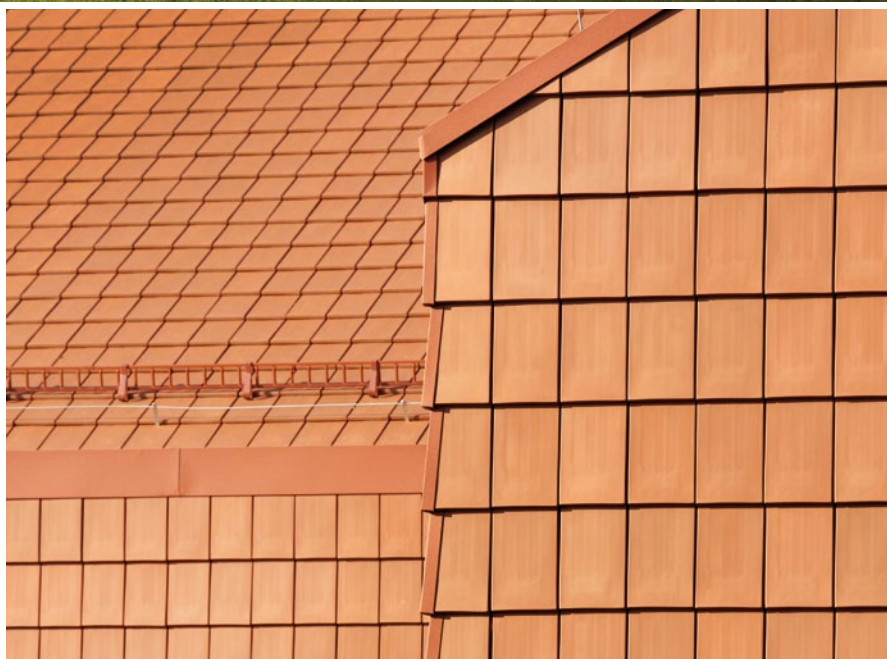
Roof and façade design creates a unified appearance: roof tiles are also ideal for façade cladding.
