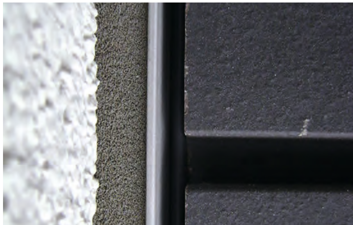
Inside corner Argeton/plaster
