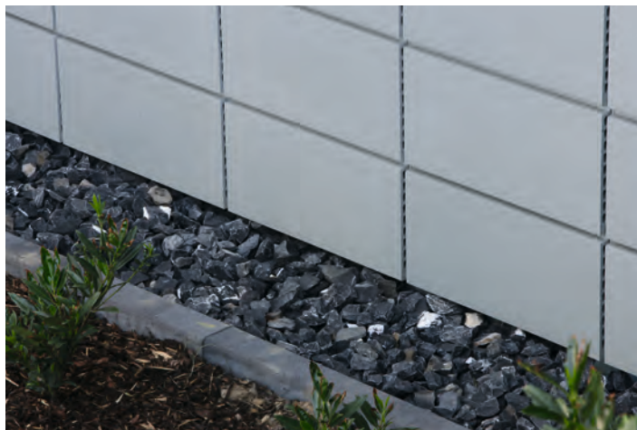
Lower finish with aluminium sheet
