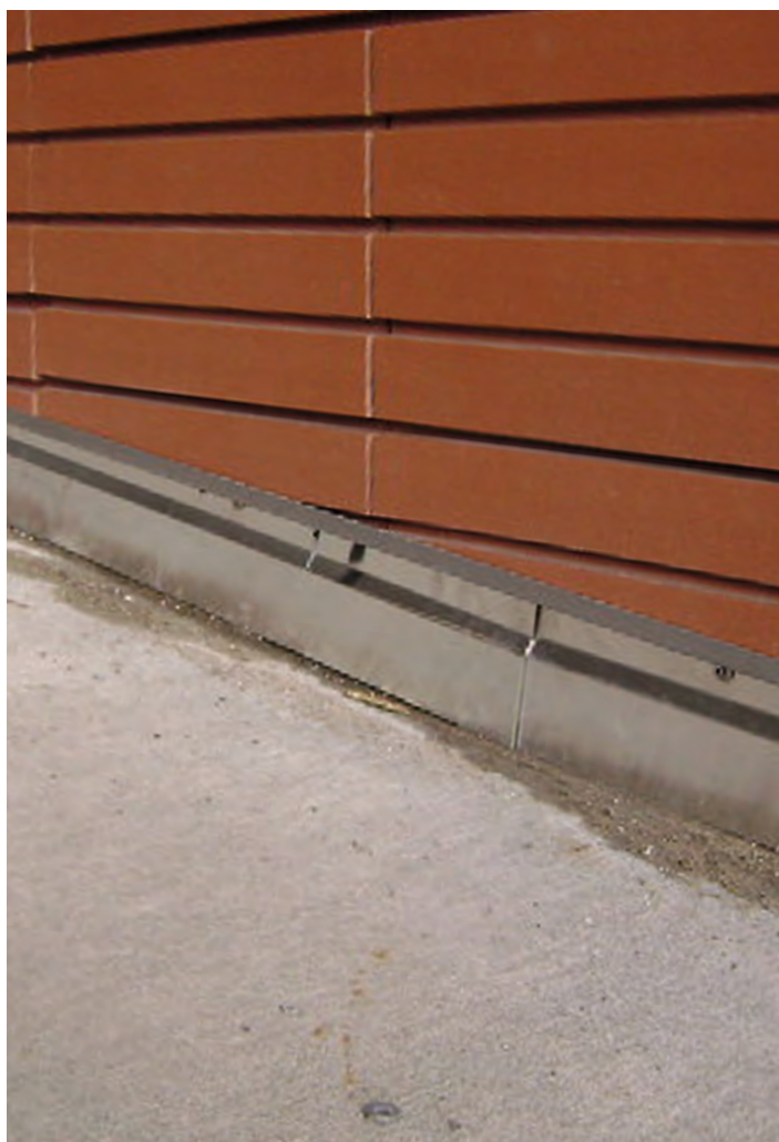
Lower finish with aluminium sheet
