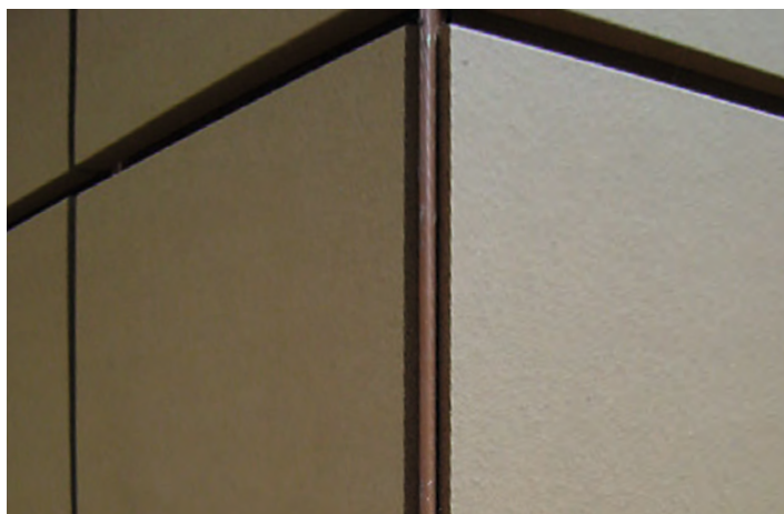
Inside corner Argeton/plaster
